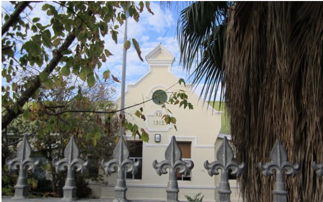
Figure 9: Brent Abrahams, "Façade of Bellville Police Station". 30 May 2016.
