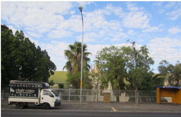
Figure 11: Bellville Police Station.
