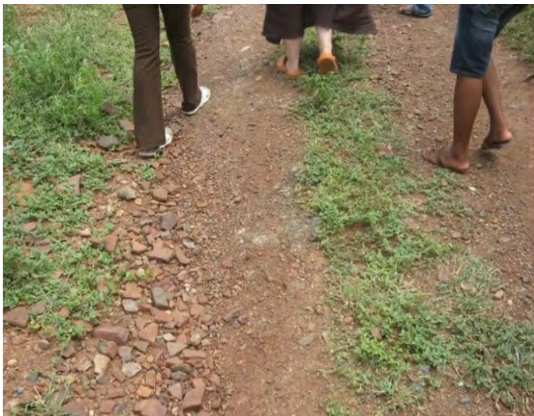
Trail with exposed asbestos, Penge, December 2008. Photo: Michal Singer
