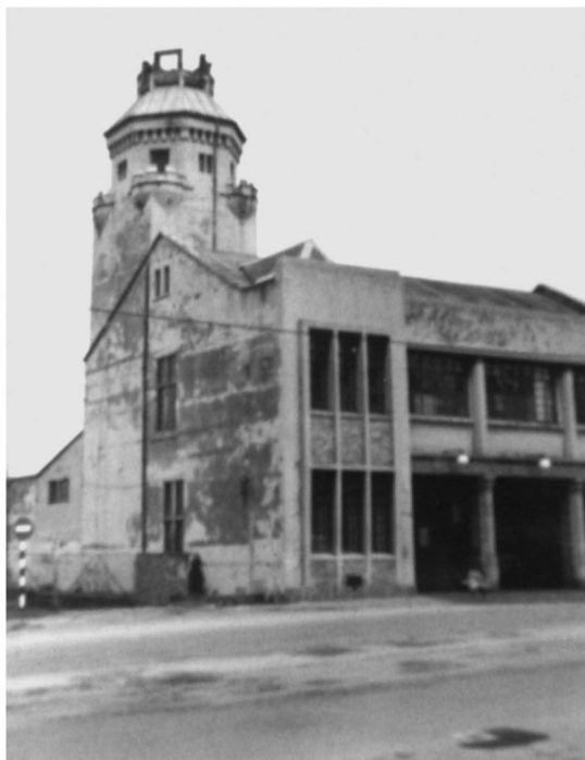
Figure 9: An East London building in decay, c. 1965.
