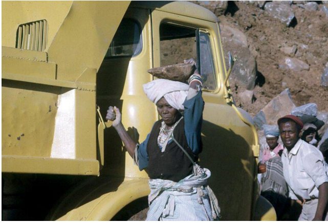
Figure 14: Construction of Tsomo Dam, 1971.
