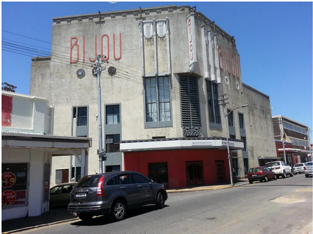
Figure 10 The Bijou building, Salt River
