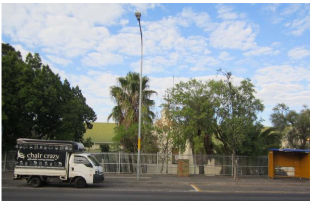
Figure 11: Bellville Police Station.
